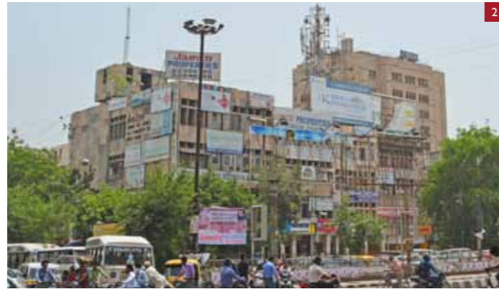
The view of the building as seen from Vikas Marg. The façade is spoilt due to random placement of hoardings and advertisement boards
