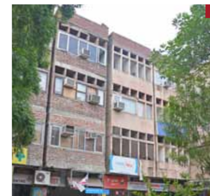
Condition of the existing façade
