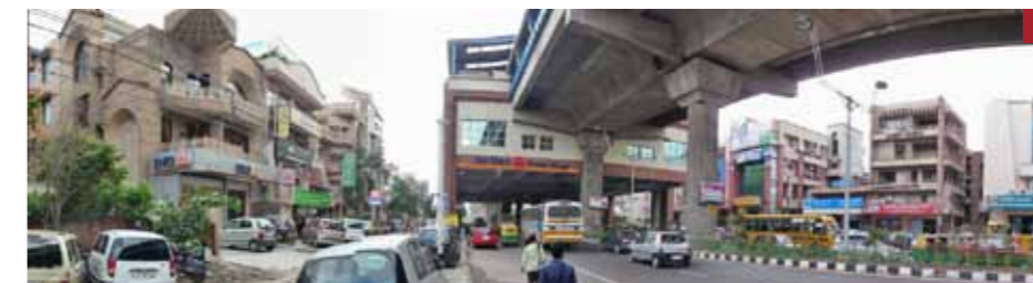
Growing Commercial Area around the Metro Station
