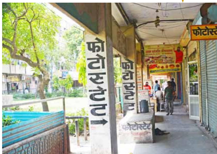
Present condition of the internal arcade
