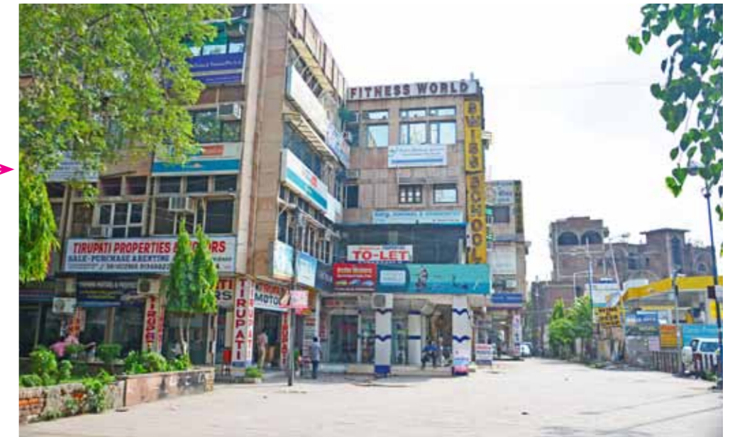
Present condition of the façade
