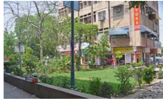
Condition of open space near CBSE building
