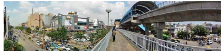
Nirman Vihar Station with the Lakshmi Nagar Commercial Complex and the adjoining V3S Mall
