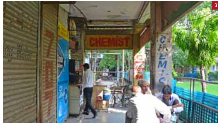
Encroached accessible corridor
