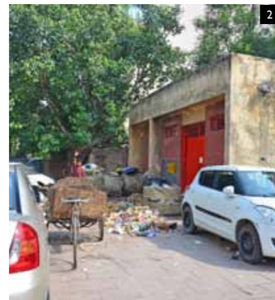
Waste dumped in front of electric substations
