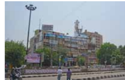
Advertising boards on the façade of the building spoil the elevation
