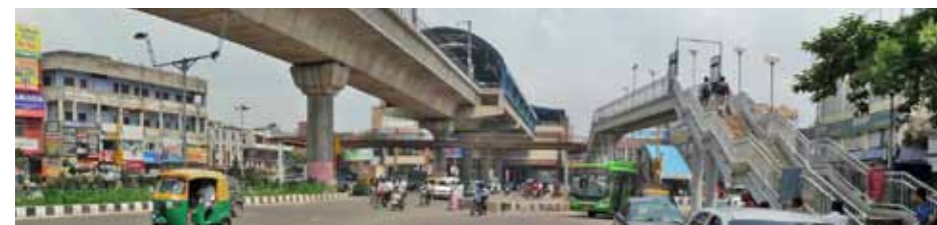
Foot over-bridges connecting Laxmi Nagar Station to different sides of the road intersection
